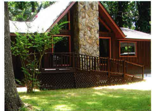
The Facility in Stone Mountain
